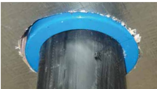
Figure 7 Penetration example - Kingspan Kooltherm® K10 FM Soffit Board installed tight around the fire collar and HDPE service pipe.
