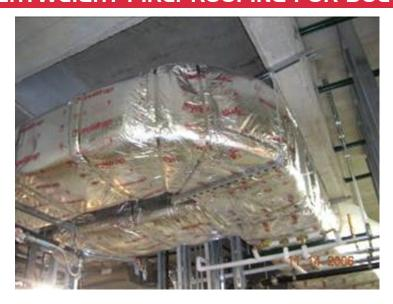
Unifrax and Trafalgar have partnered in Australia to bring you FYREWRAP duct fireproofing systems. Simply put, this is the only way to go when it comes to providing passive fire protection for ductwork in commercial buildings.
