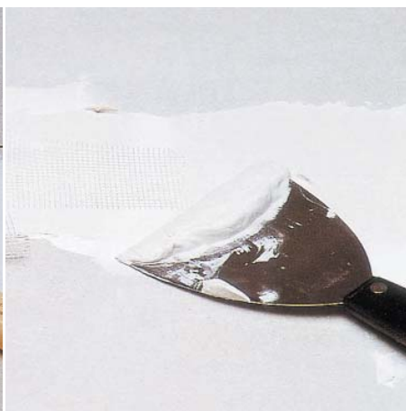
Skim coating the board joint.
